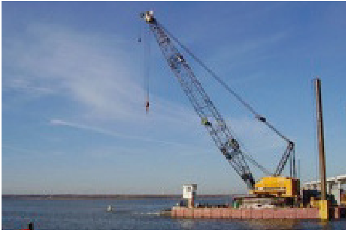
Typical portable land crane on raft of flexifloats
